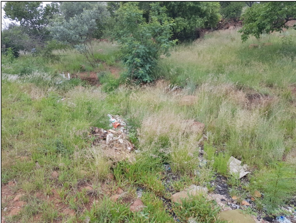
Photograph 4: Uncontrolled fill material ( Photograph taken near test pit TP05 in a NE direction )
