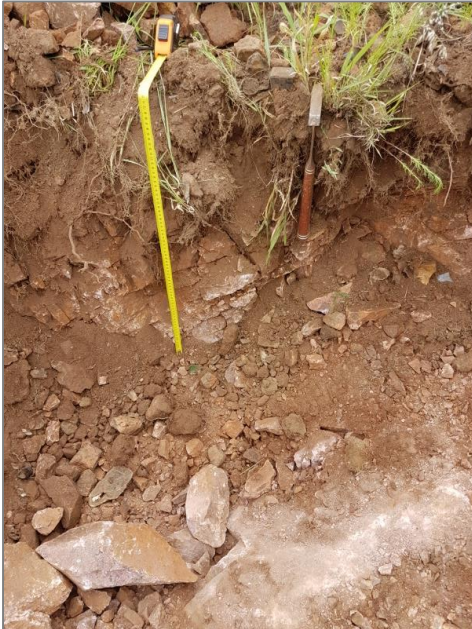
Test Pit no: TP06
